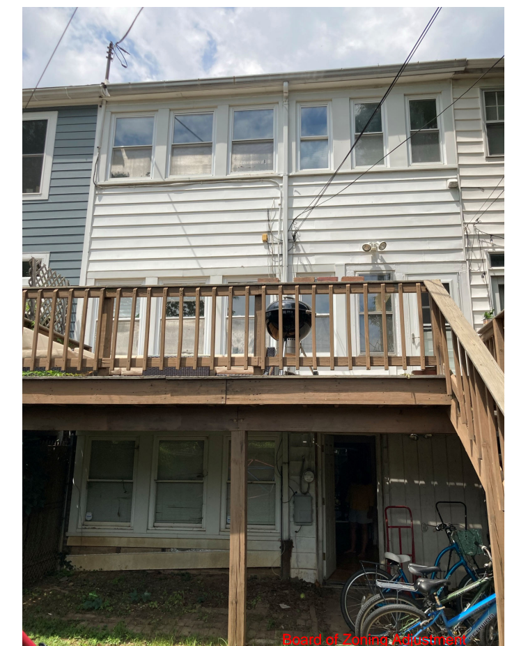
EXISTING REAR FACADE
